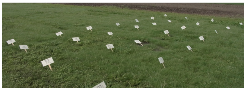
Picture 4. Experimental plots at the John Seaton Anderson Turf and Ornamental Research Facility at Mead, NE. Safety and efficacy of 13 herbicides applied at zero, two or four weeks after seeding of Sundancer buffalograss were evaluated in 2012 and 2013. Photographed in August, 2013.
